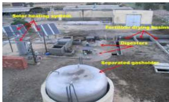
Fig. (\*\*): biogas and bio-fertilizer production system
